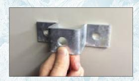
2. Drill Holes where marked for fixings suitable for wall material (PLEASE NOTE,: we do not supply screws or anchor bolts as we cannot specify the type of wall material the sign will be fixed to).
